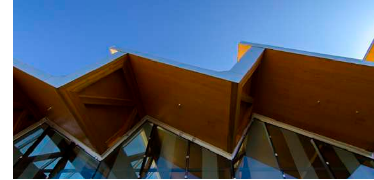
■ Skylight truss overhang, AMS Student Nest
