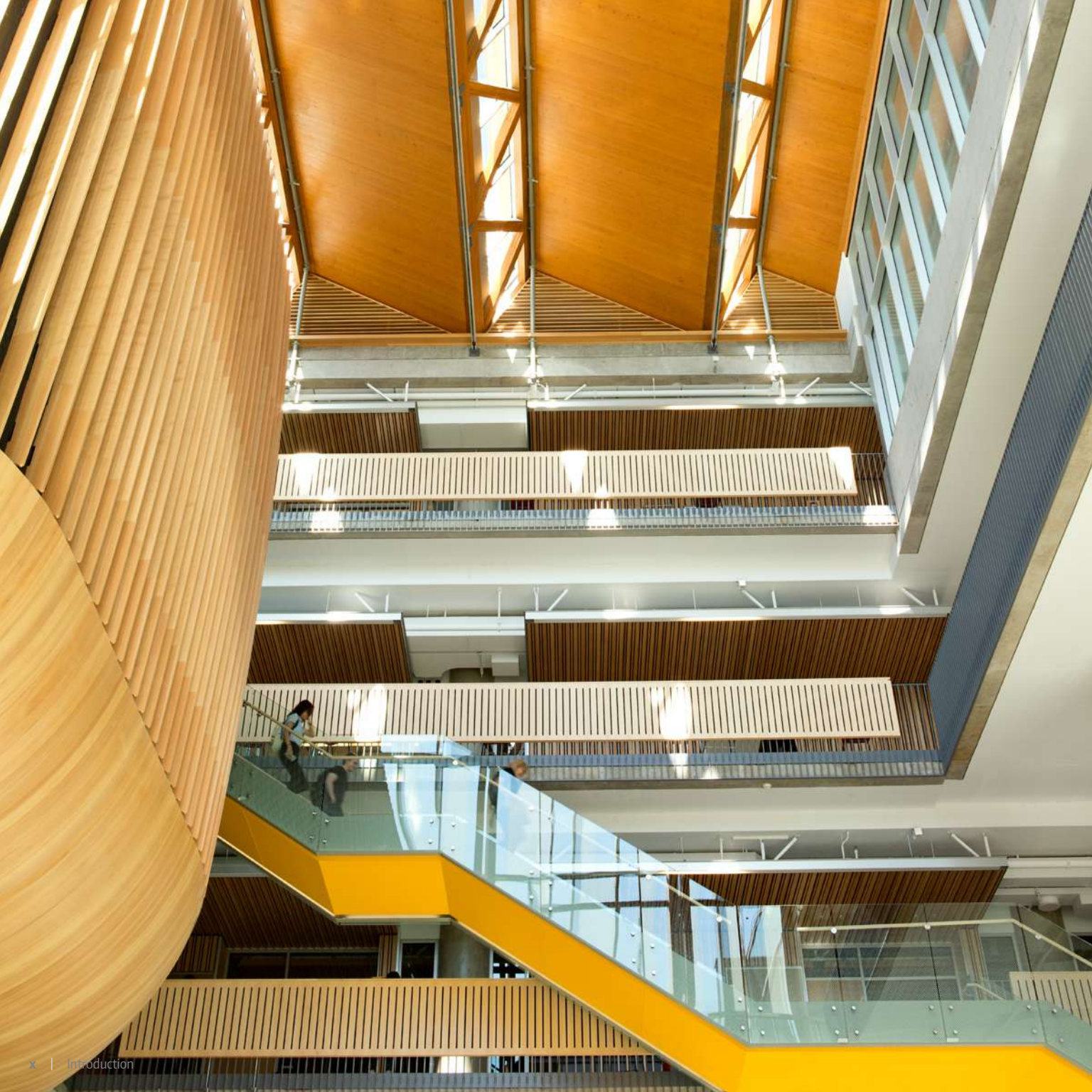
Looking up through the Agora to the Cross-Laminated Timber skylights in the AMS Student Nest
